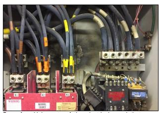
One of multiple parts of the electrical panel that were burned out by the electrical surge.
