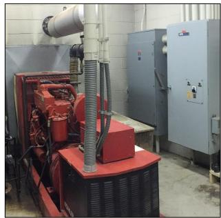
Diesel generator and electrical panel damaged by the storm.
