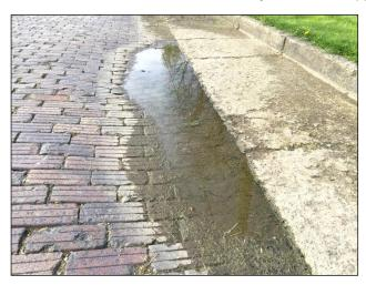
The project will replace the concrete curbs and gutters, plus replace storm water catch basins. The existing curbs and gutters are generally in poor condition and there are several locations where storm water stagnates instead of draining away properly.
