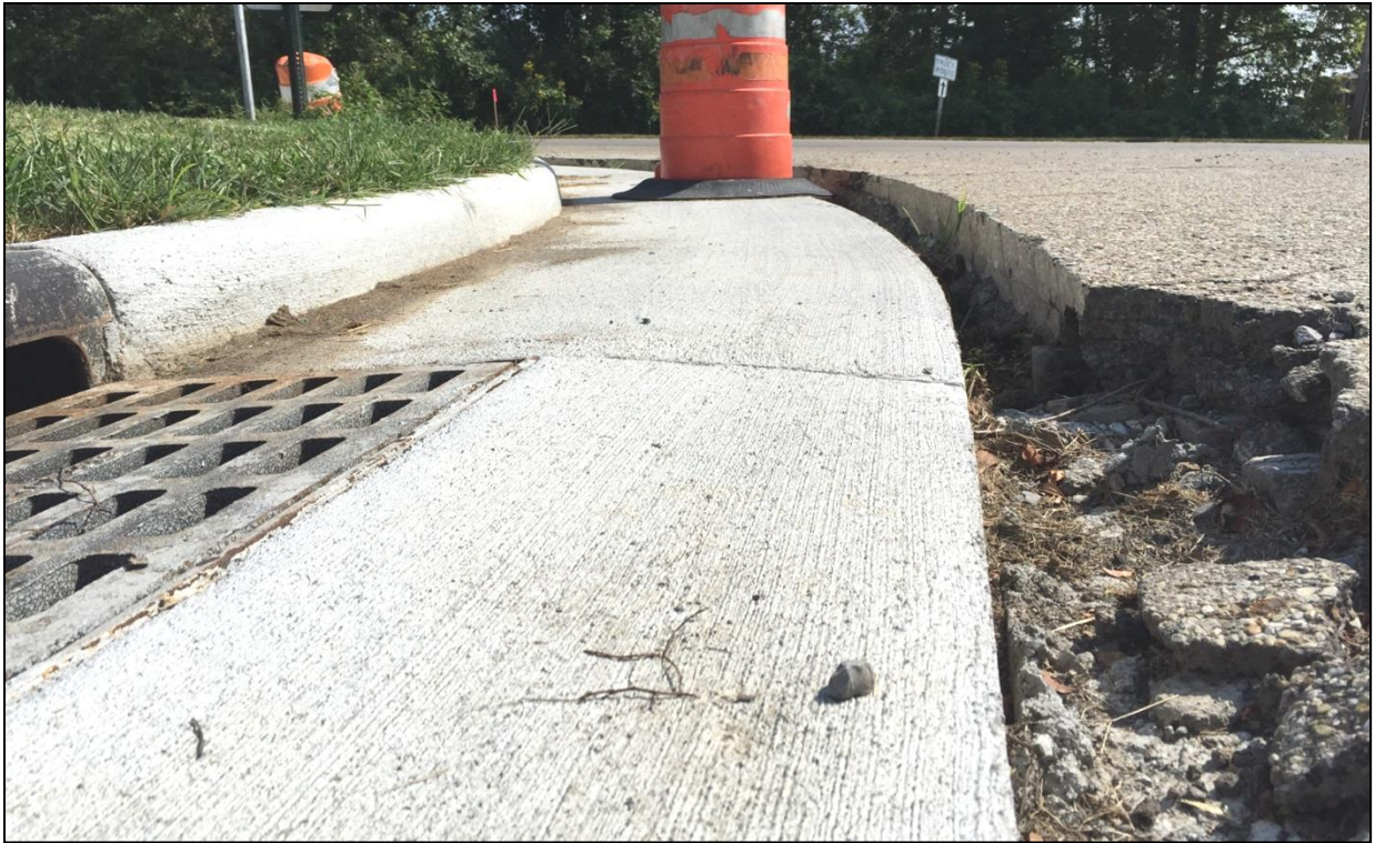
Detail of pavement and gutter on the east side of Strayer Avenue
