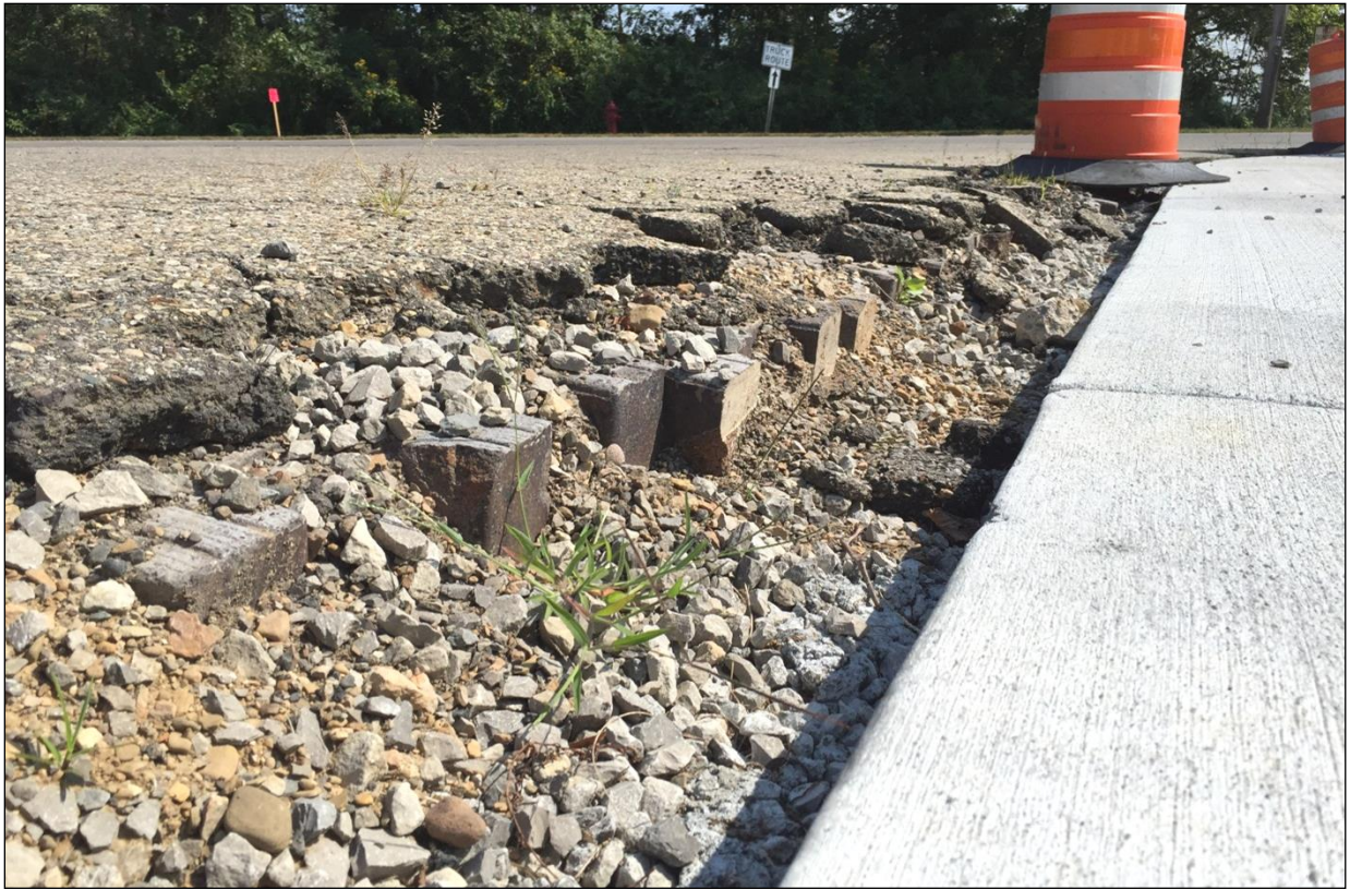
Detail of pavement and gutter on the west side of Strayer Avenue
