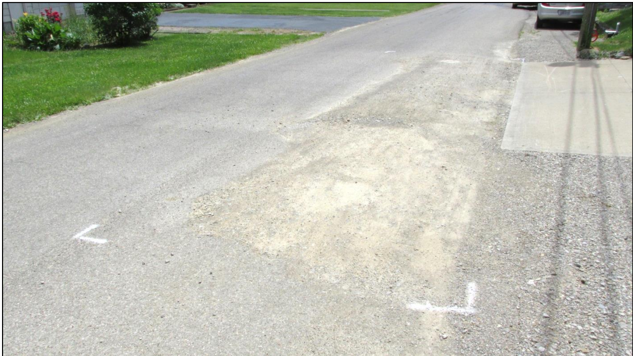
Site of a water main break repair during Winter 2015-2016.
