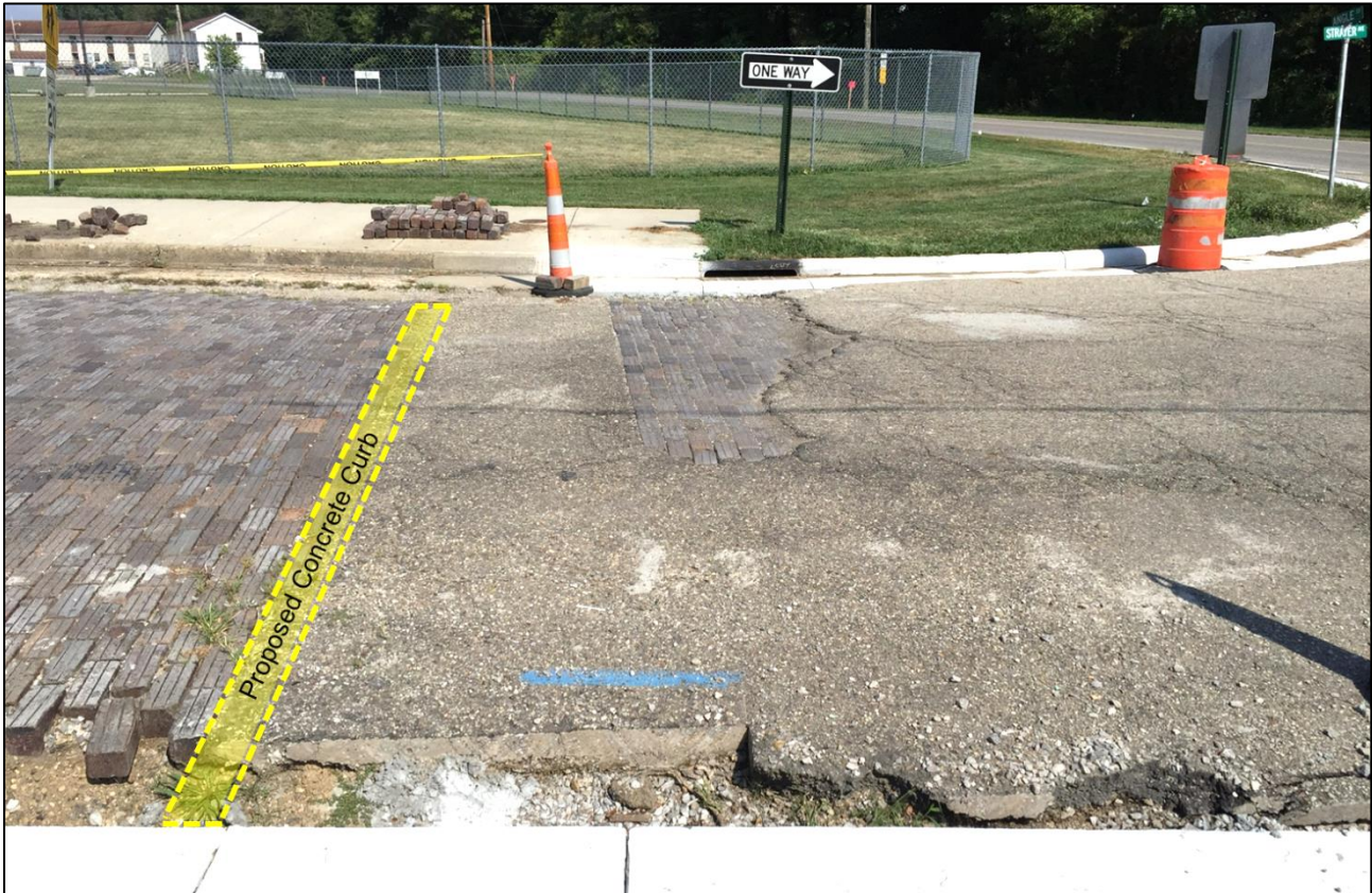
A concrete divider curb will be installed at the south end of Strayer Avenue, by Village crews, to establish a defined separation between brick and asphalt pavements. This will be completed prior to the asphalt pavement repairs.
