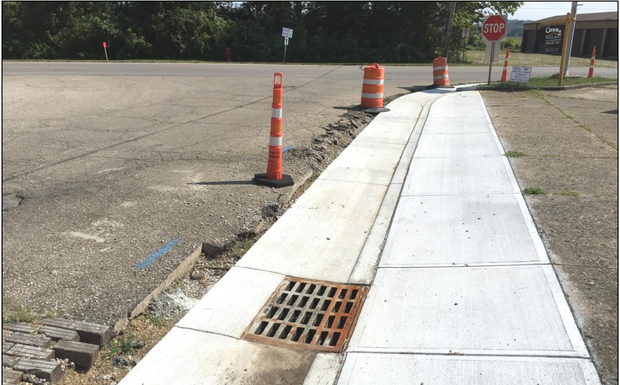
Overview of the west side of Strayer Avenue
