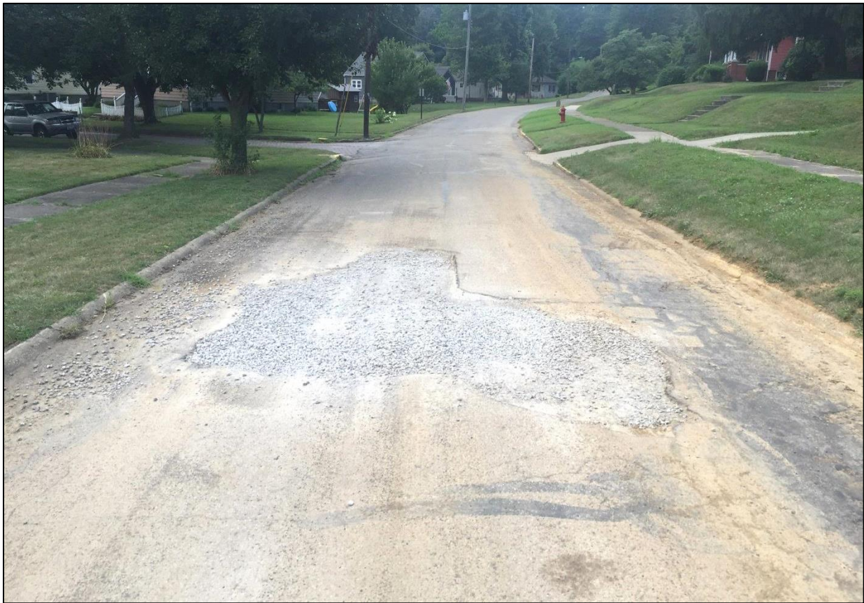
Site of a sinkhole repair, July 2016.
