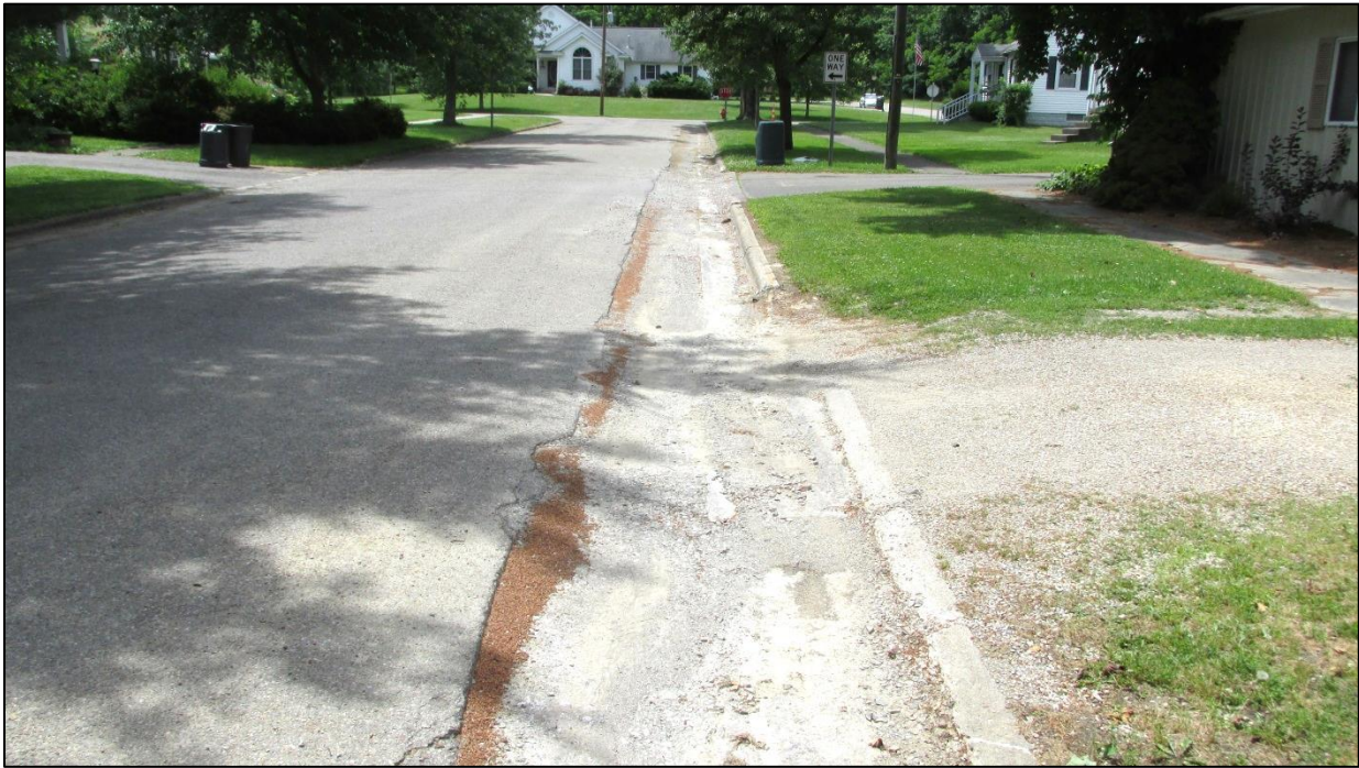
Site of storm sewer pipeline installation on Maple Street connecting storm catch basins on School Street and Bartlett Street.
